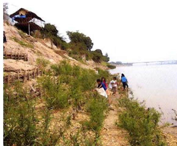
Simple Vegetation Riverbank Protection & Greening Work by Planting Mekong Willow
